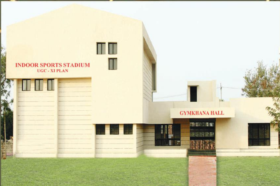
Indoor Sports Stadium
